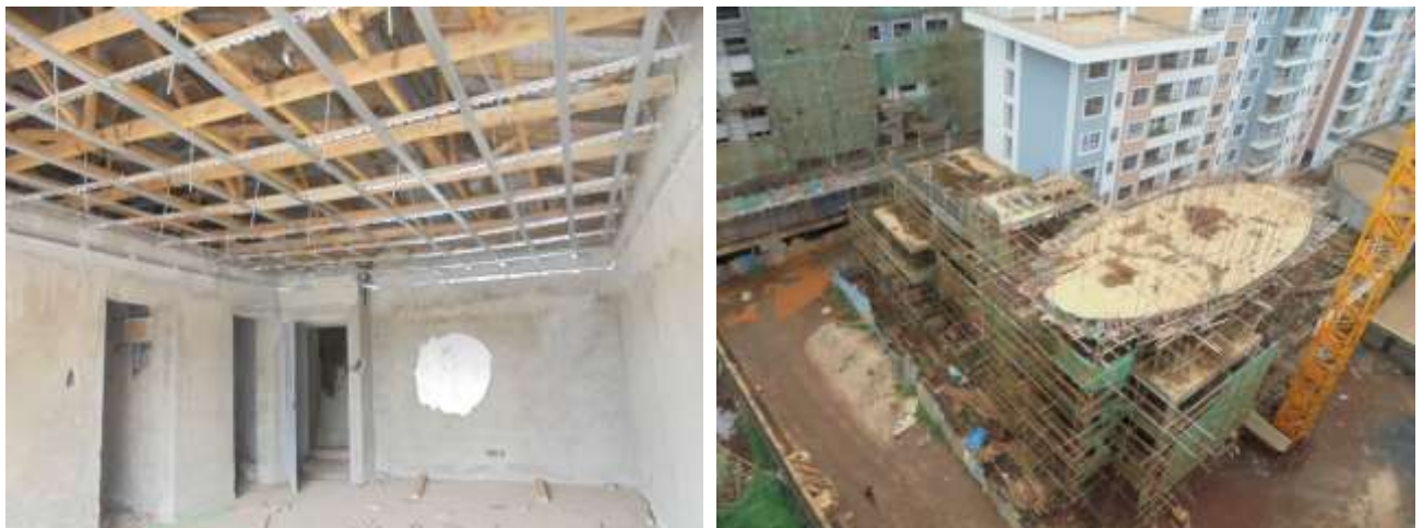
-Some of the pending works-
